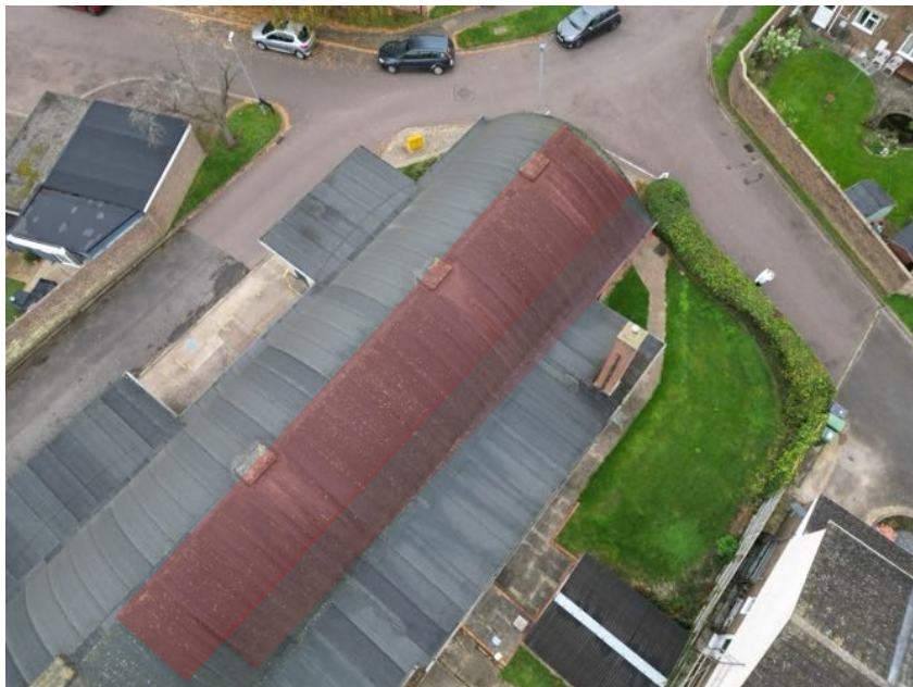
Photo showing left hand side roof slope (shaded in red) which displays a high level or surface lichen growth
