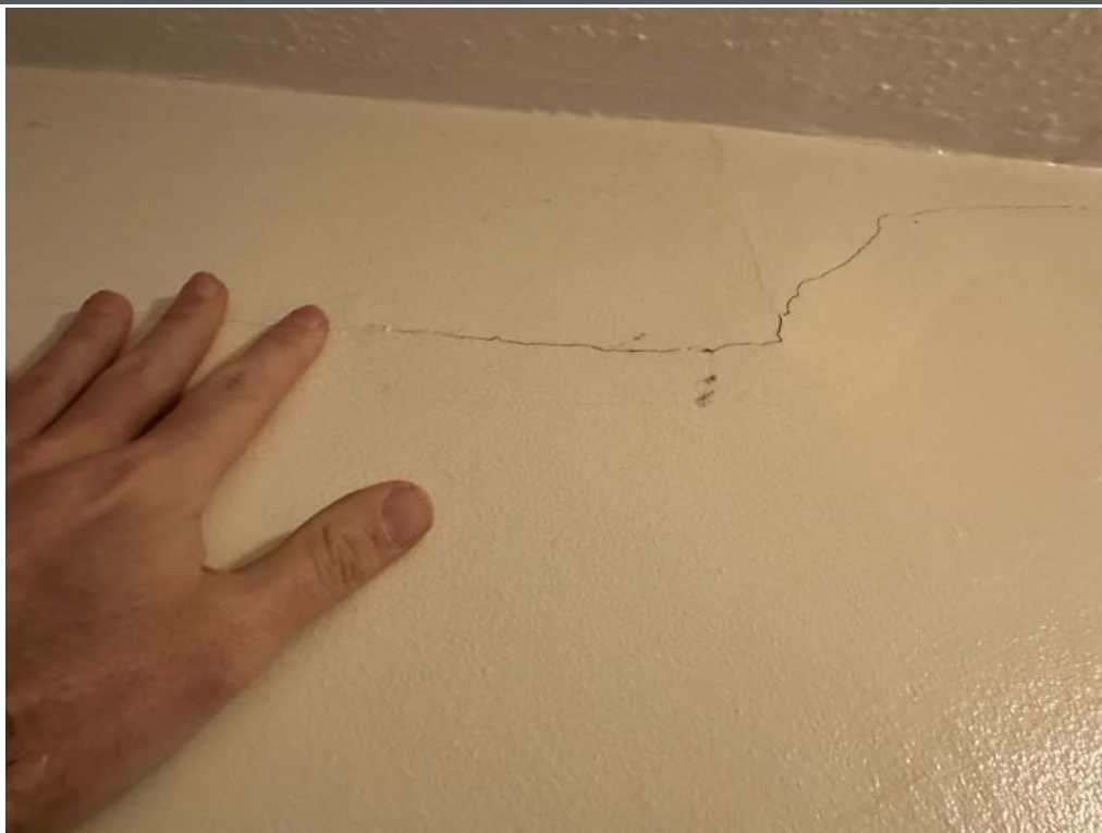
Photo showing cracking pattern which is showing either side of the arch through to the Hallway.
