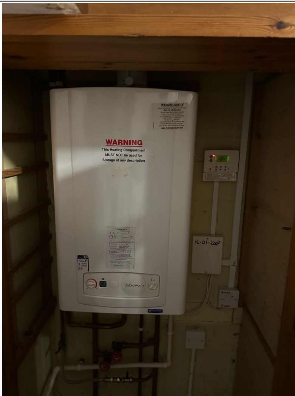
Photo showing Glow Worm Boiler which was clearly operable at the time of our visit.
