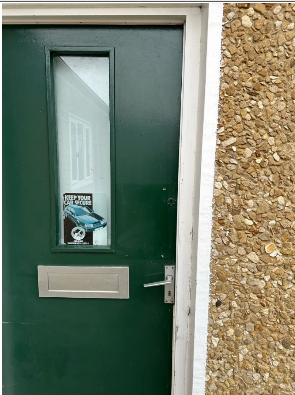
Photo showing door into the side store – note that we do not believe the glazing to this vision panel to be toughened glass. This could lead to break in or injury.
