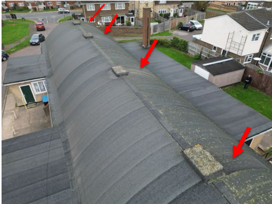
Photo showing raised vents which are providing a cross flow of ventilation to the roof
