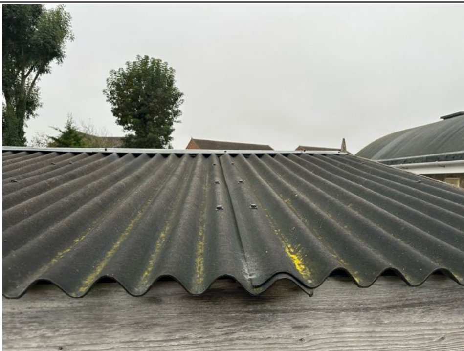
Photo showing Onduline bitumen fibre roofing showed no signs of significant undulation
