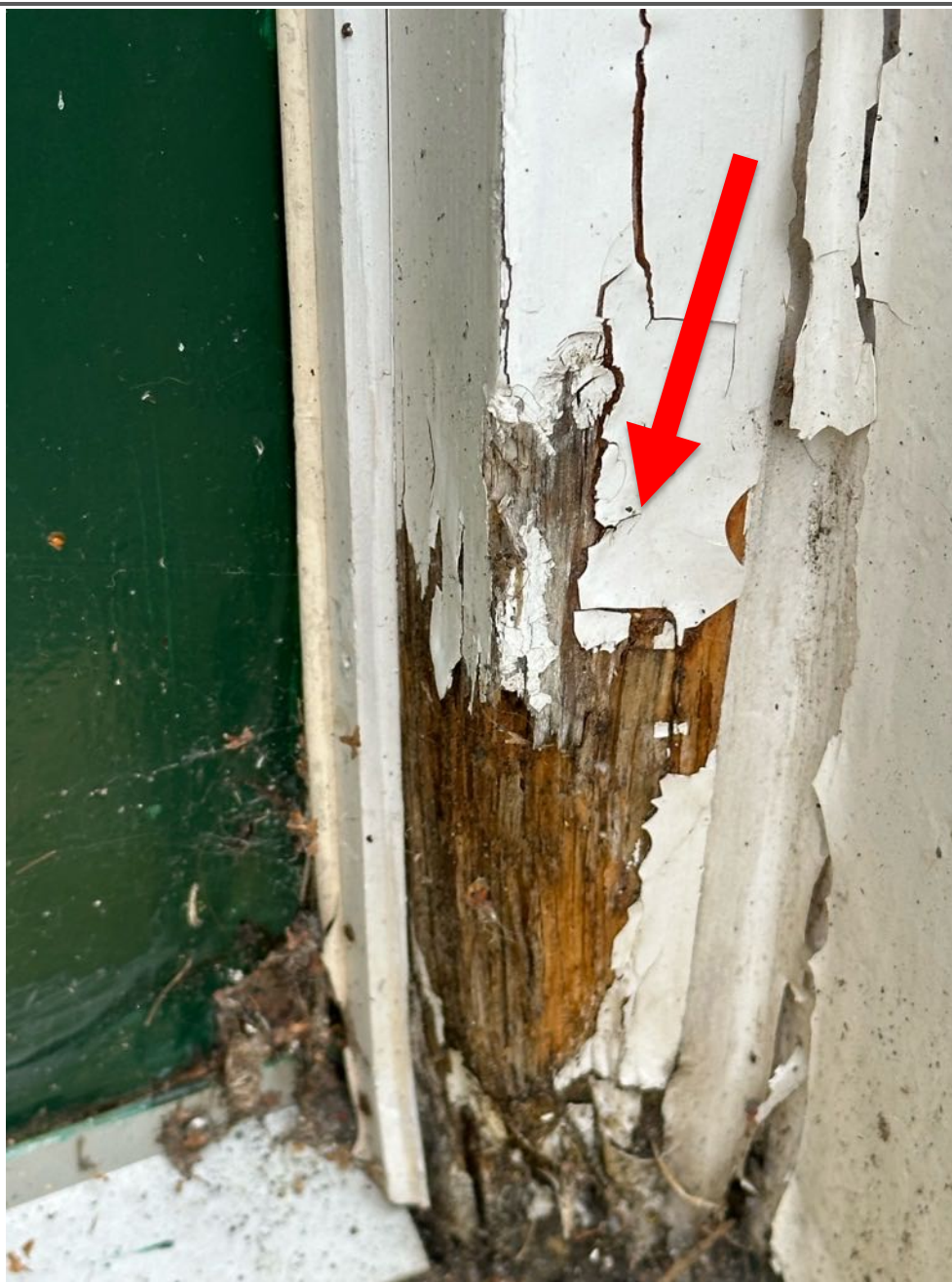
Photo showing timber decay to the door surround to the side store. We would suggest cutting out these areas of rot and splicing in new sections of timber.
