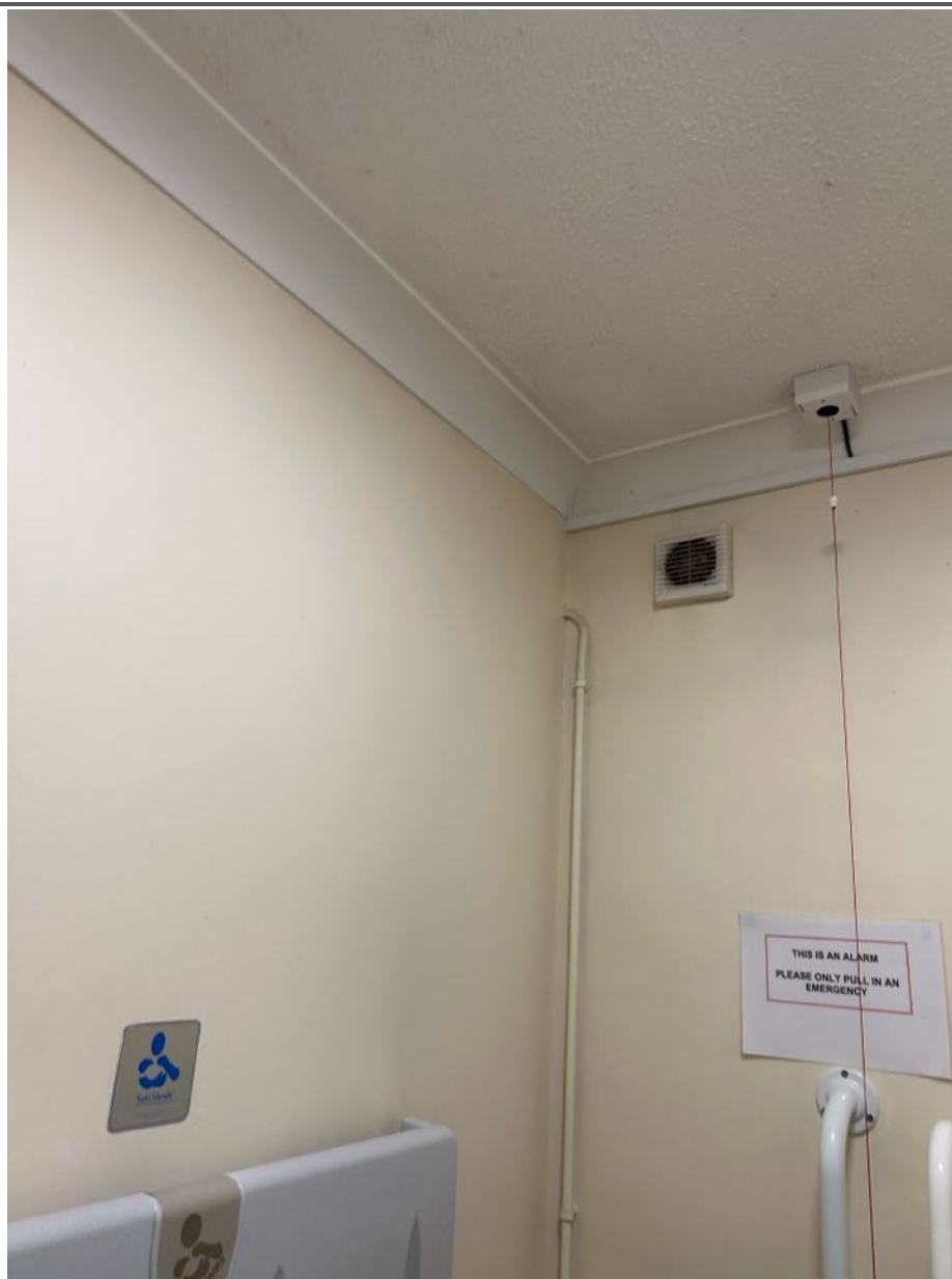
Photo showing mechanical extraction to the WC which was operable at the time of our visit
