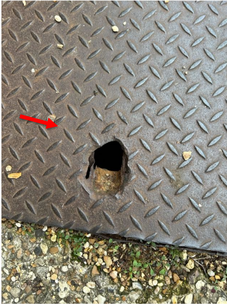
Photo showing damage to the steel inspection
