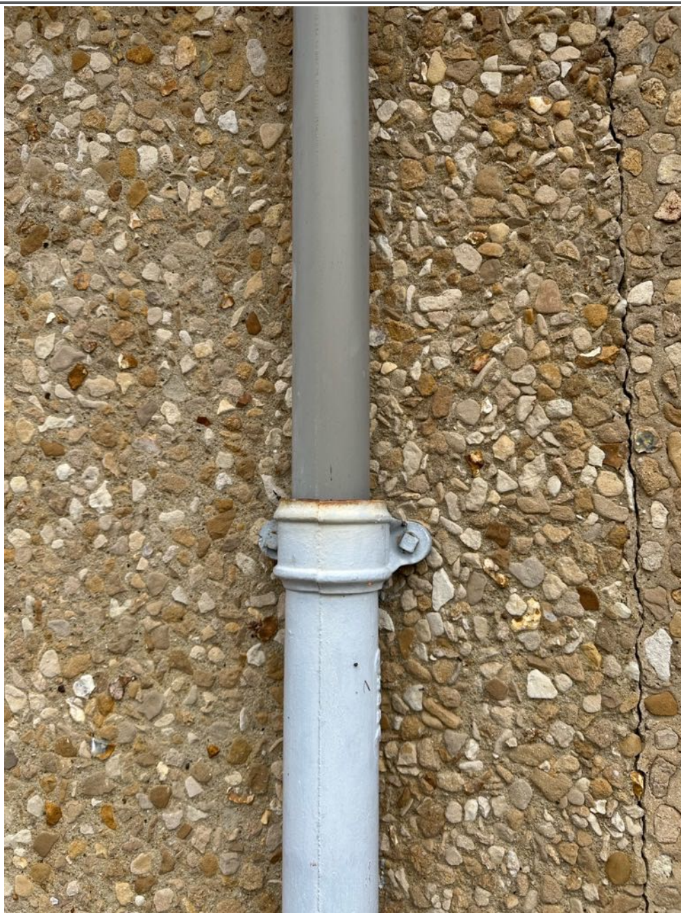
Photo showing plastic guttering discharging into cast Iron section of downpipe
