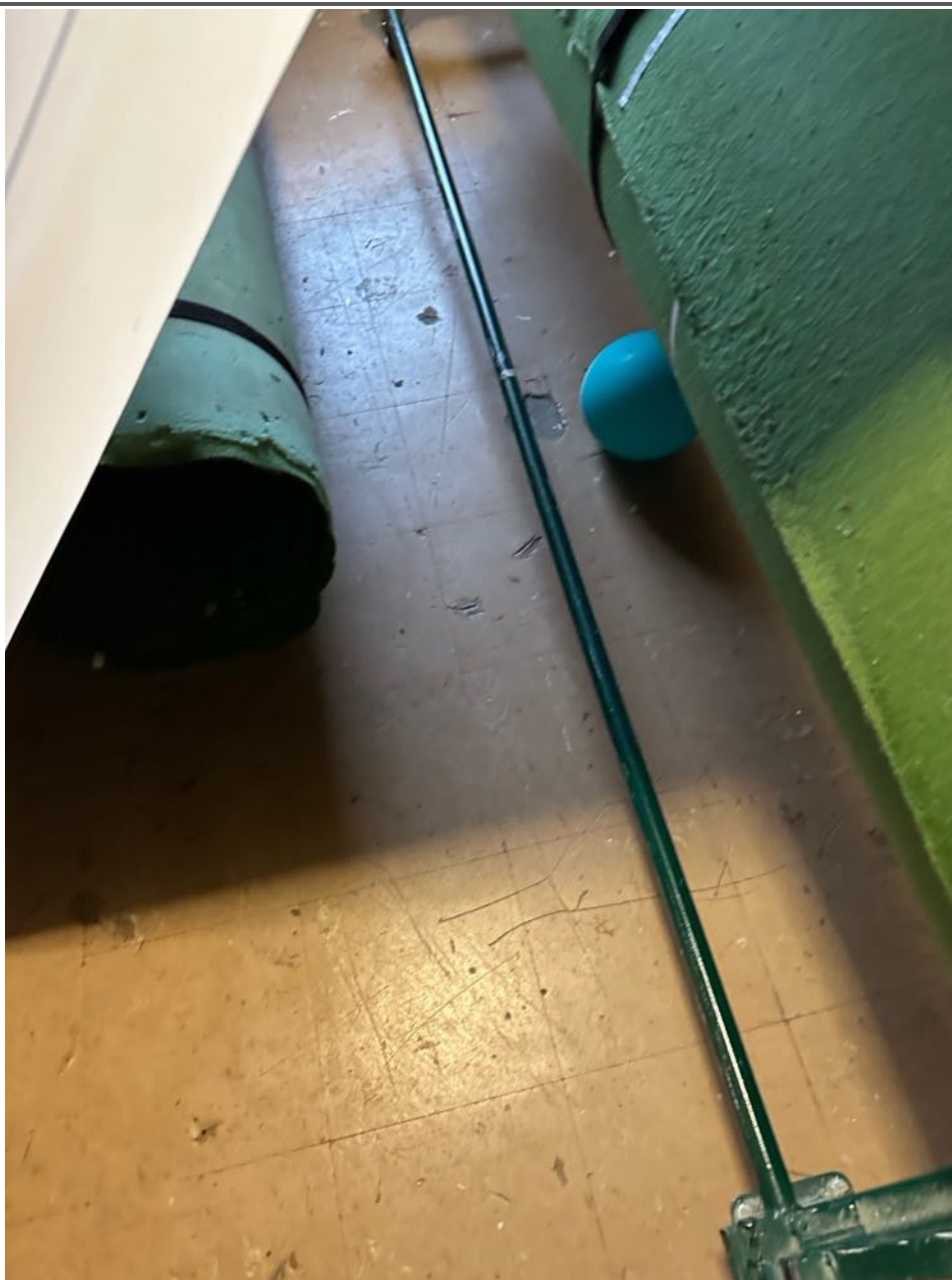
Photo showing generally poor condition of the thermoplastic floor tiles with numerous chips noted
