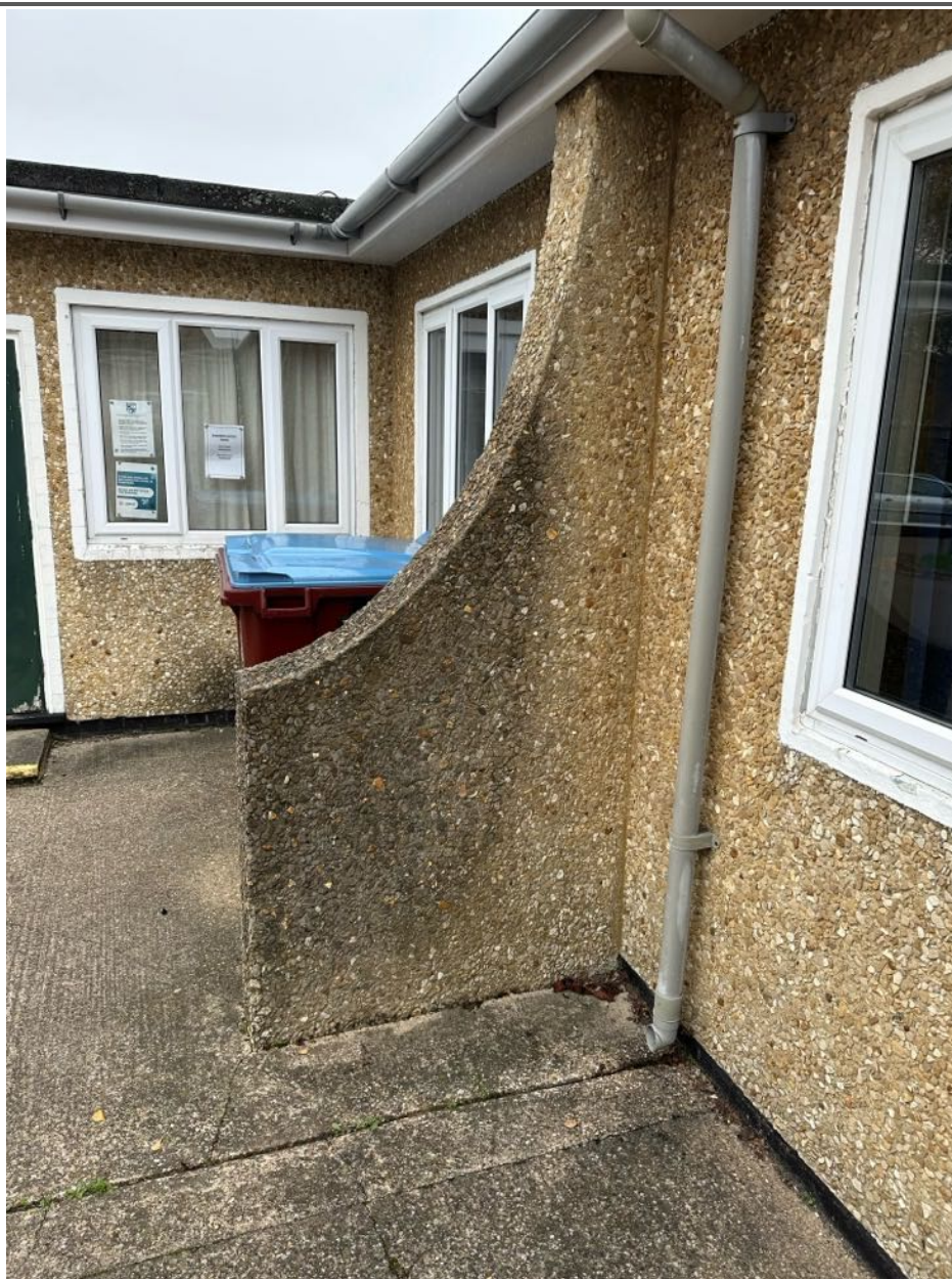
Photo showing concrete buttress to the right hand side which is providing lateral restraint to the walls
