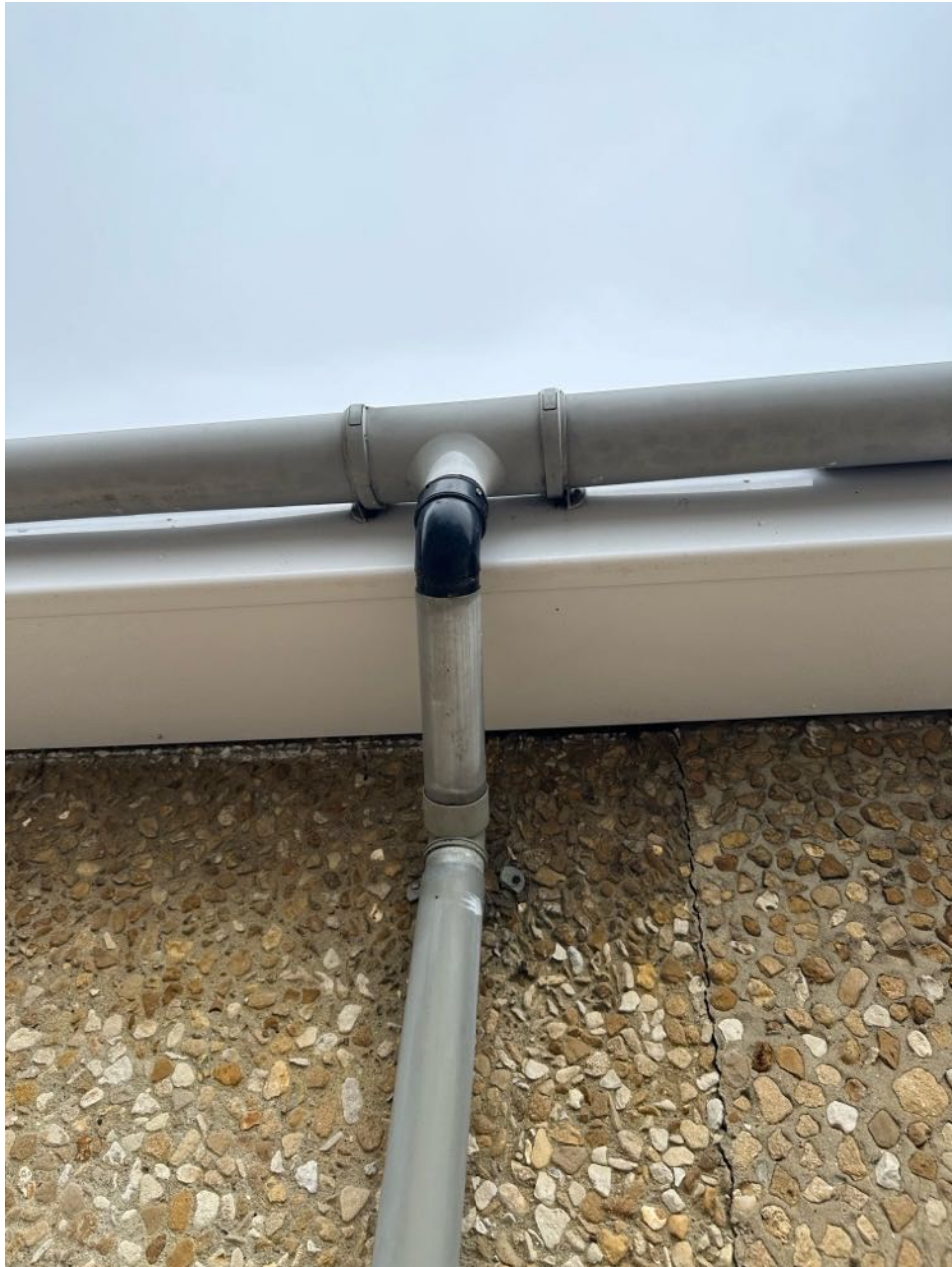
Photo showing mis matched type of guttering with plastic gutters, aluminium sections and lined down pipes. Note that the gutter clips are broken.
