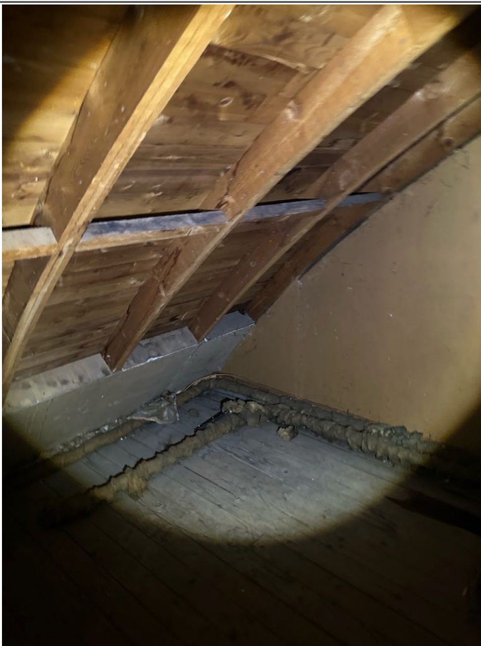
Photo showing timber sarking board on curved timber rafters internally
