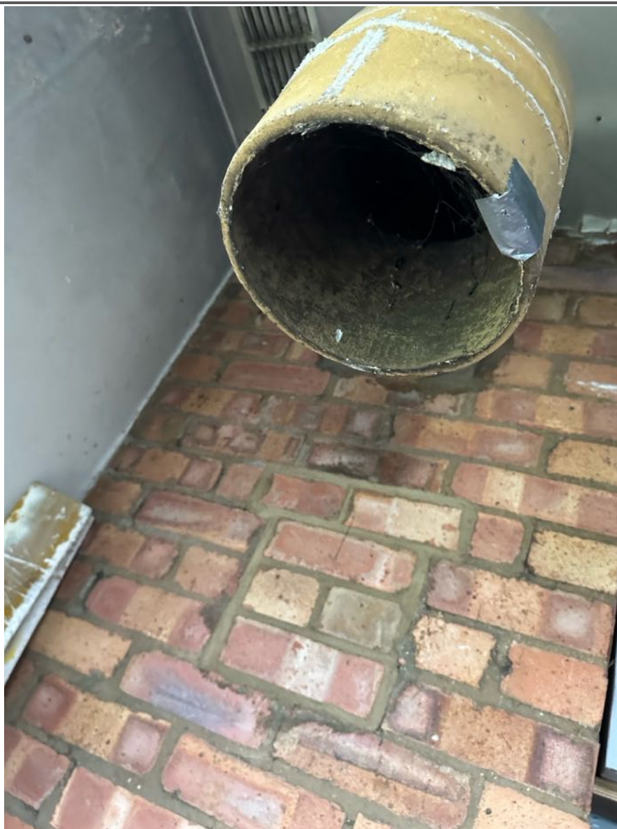
Photo showing potentially Asbestos containing flue product to the boiler room which we believe is connected to the chimney above
