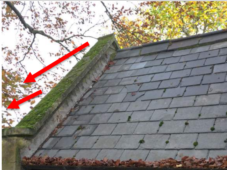
Photo showing bowing of the gable end wall which has clearly been occurring
