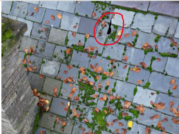
Photo showing damage to the chapel roof where we believe Water is entering the roof
