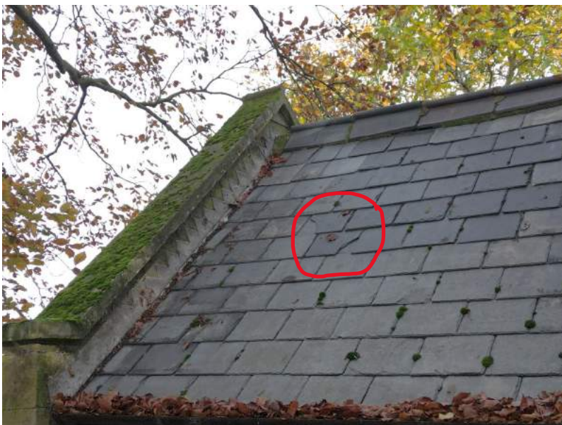
Photo showing cracked and damaged slates
