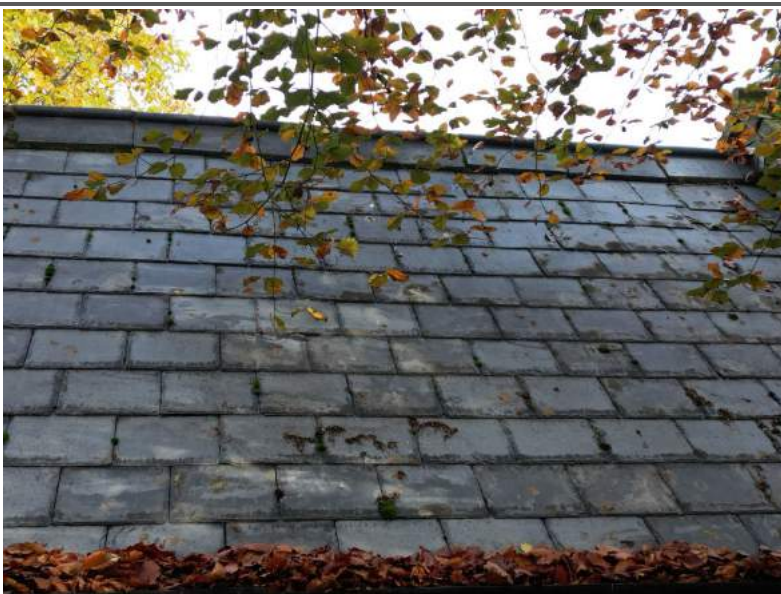
Photo showing cracked and damaged slates
