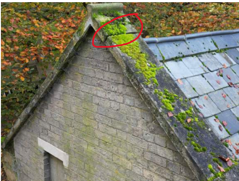
Photo showing Gapping to the coping to the gable end
