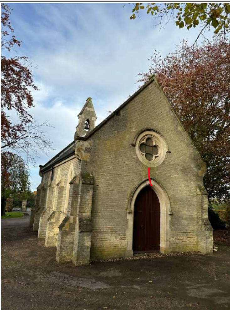
Photo showing cracking over the rear door arch
