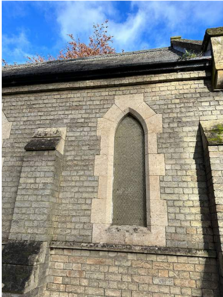
Photo showing glass reinforced plastic window
