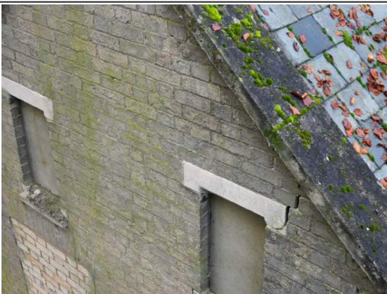
Photo showing failed lintel over the right hand gable end window
