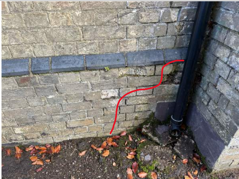
Photo showing area of washed out mortar to brick joints
