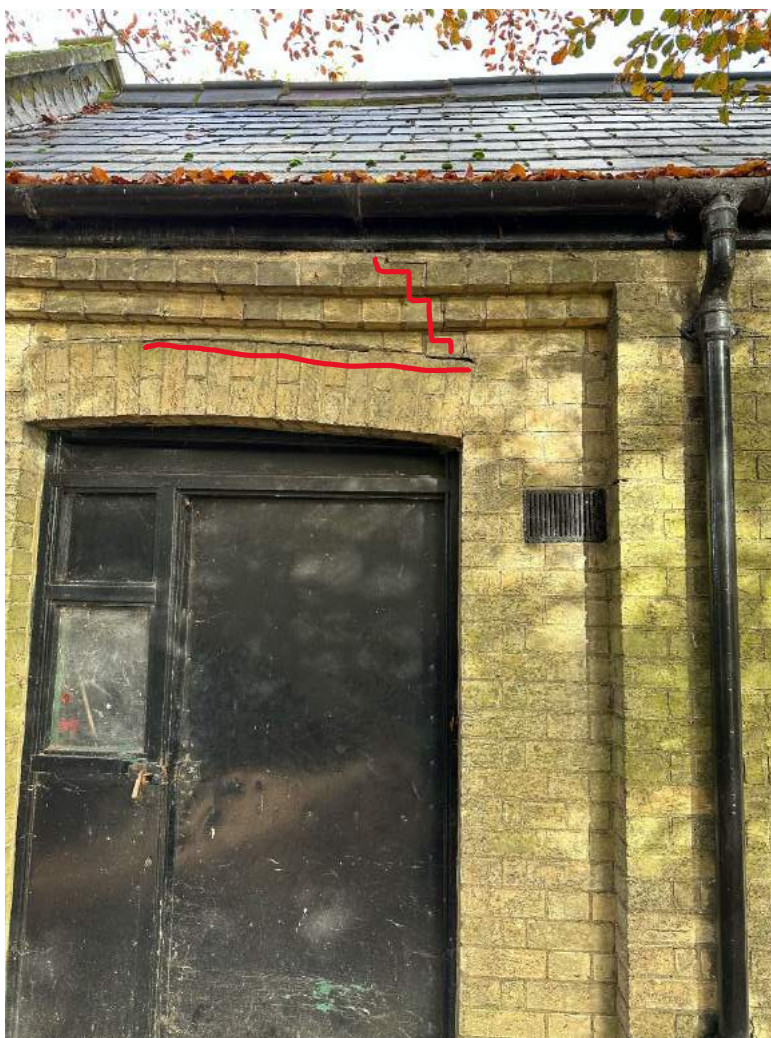
Photo showing dropped lintel over door head in need of repair
