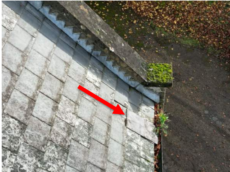
Photo showing slipped slate and blockage within the gutter
